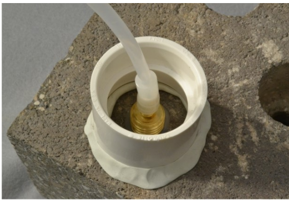
Figure 6. Water dam used for leak detection.
