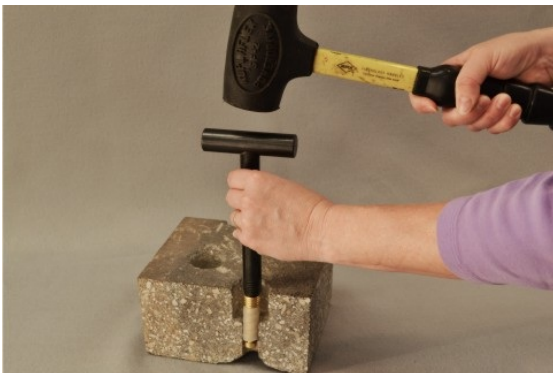
Figure 3. Flush-mount installation.
