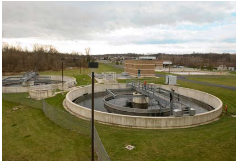
Food, swimming pools, wastewater and aquaculture are typical sampling applications for the ORP15 pen.
